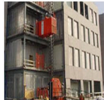
Typical Construction Hoist
